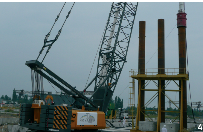
August 2010: Driving the metal piles for the longitudinal beams in the assembly area.
