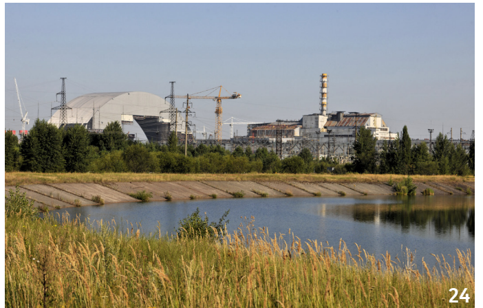
August 2014: Second lifting operation for the second half of the arch. ©Francis Vigouroux
