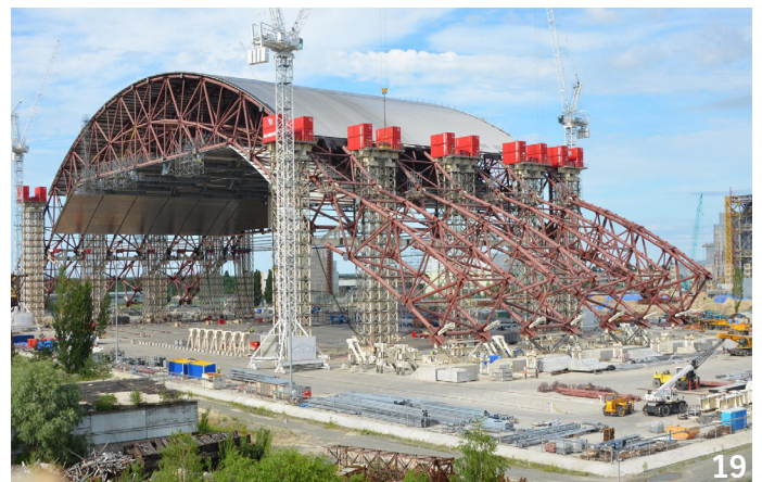
June 2013: Second lifting operation.
