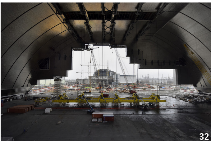
November 2015: Lifting the first overhead bridge cranes inside the arch. ©Francis Vigouroux
