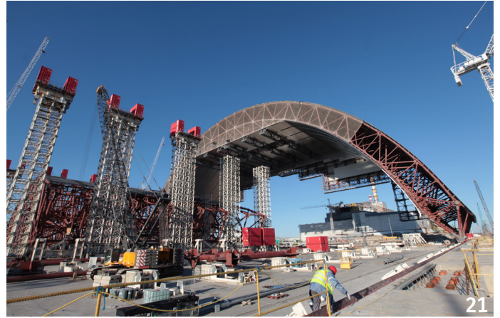
April 2014: First half of the arch pushed to the waiting position (4) and first lifting operation for the second half.
