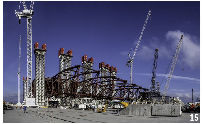
November 2012: First arch lifting operation. - @Jean-Yves Govin Sorel
